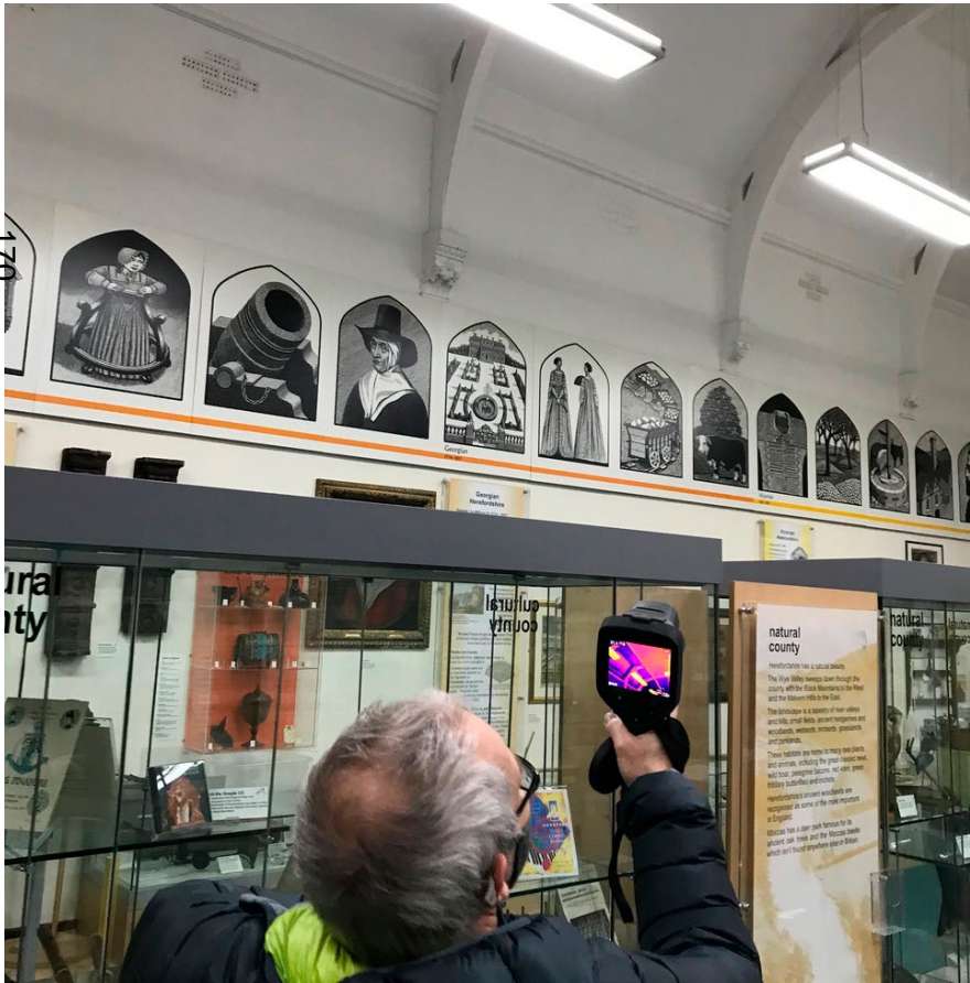
Fig. 91 / Forensic Investigation / Thermography camera highlights original roof lights in Museum space. Source: Archetype, 2021.
